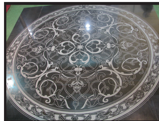
Marble Floor Tiles engraved with a laser.
